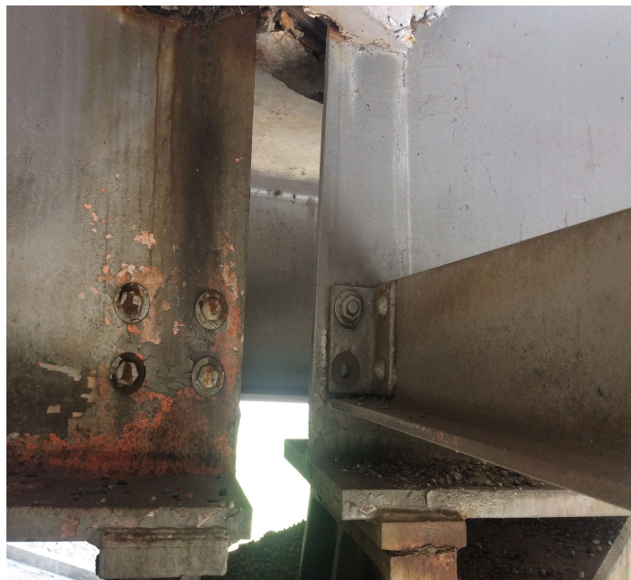
PHOTO 1 Description Bent 2 girder 4 has 2 missing bolts in bottom of diaphragm connection.
