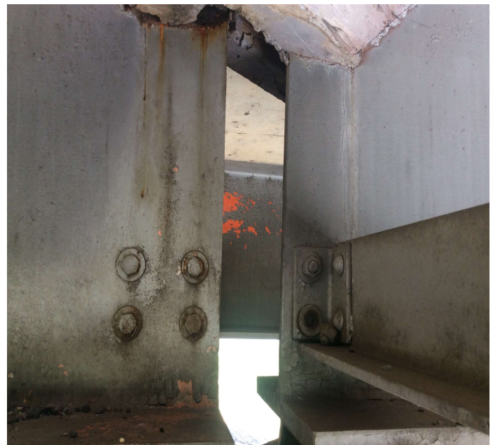
PHOTO 2 Description Bent 2 girder 5 has 1 sheared bolt in diaphragm connection.
