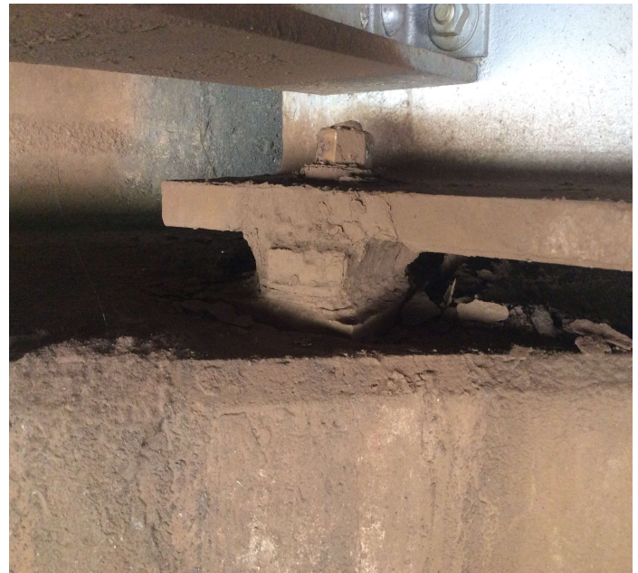
PHOTO 2 Description Bent 4 girder 3 and 4 have floating bearings.
