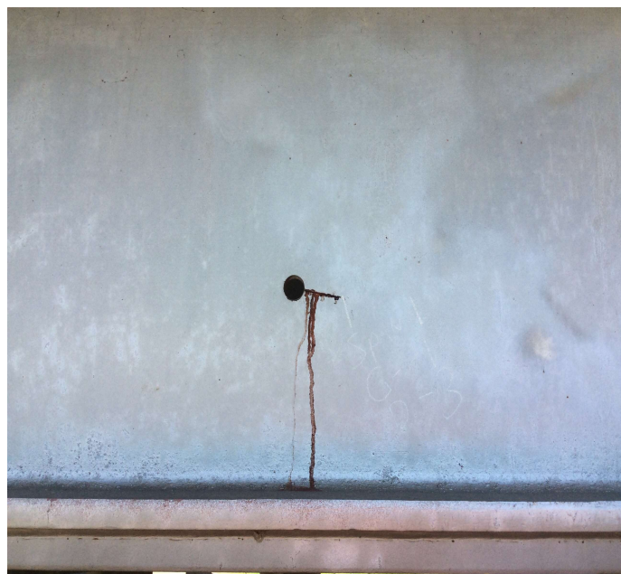
PHOTO 5 Description Span 1 girder 1 diaphragm 3 crack in web.
