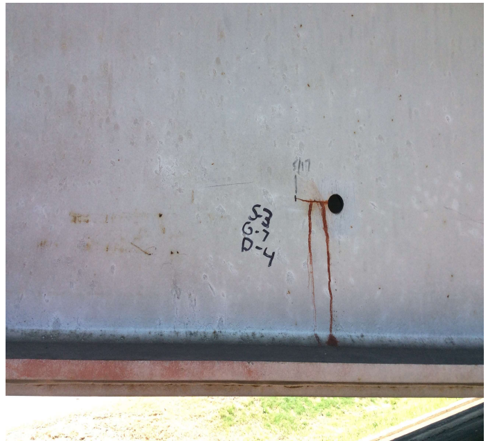
PHOTO 2 Description Span 3 girder 7 diaphragm 4 crack in web.
