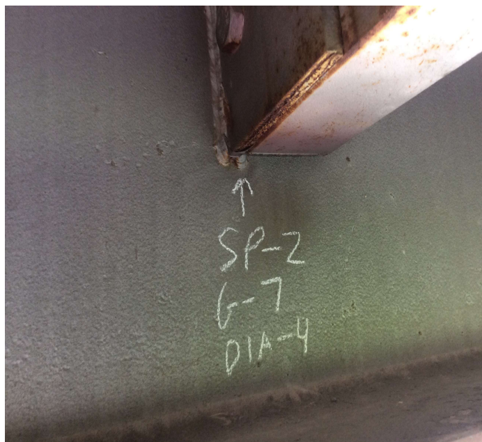
PHOTO 3 Description Span 2 girder 7 diaphragm 4 crack in toe of weld.
