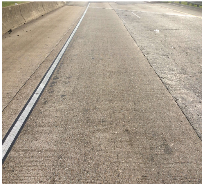
PHOTO 2 Description Longitudinal cracks in span 3.
