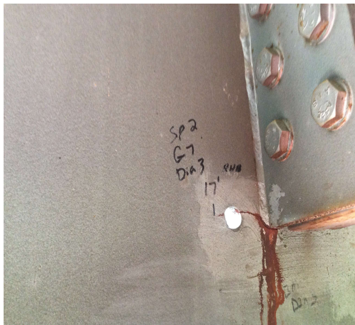
PHOTO 4 Description Span 2 girder 7 diaphragm 3 crack has propagated out of arrest hole into web.
