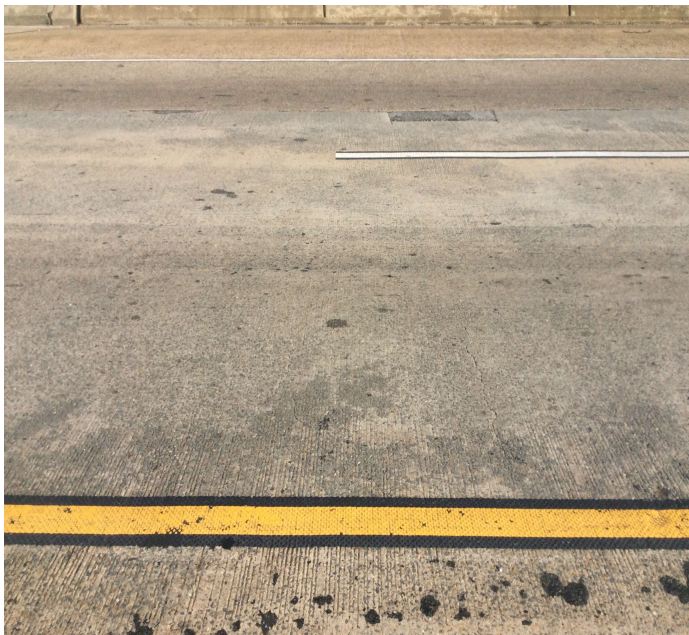
PHOTO 1 Description Transverse cracks in span 1 left lane.
