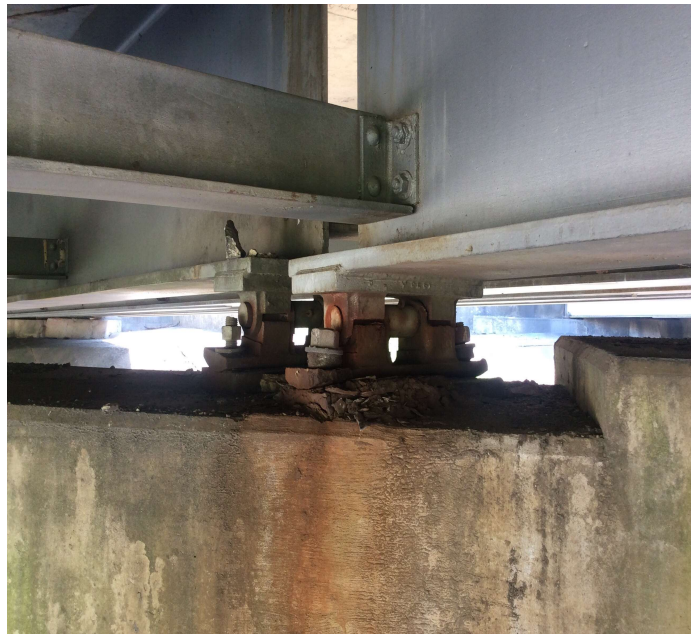
PHOTO 1 Description Bent 3 bearing 4 pack rust.
